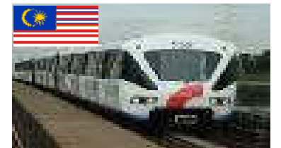
LRT Package B Completed : 2015 Value: RM569mil
