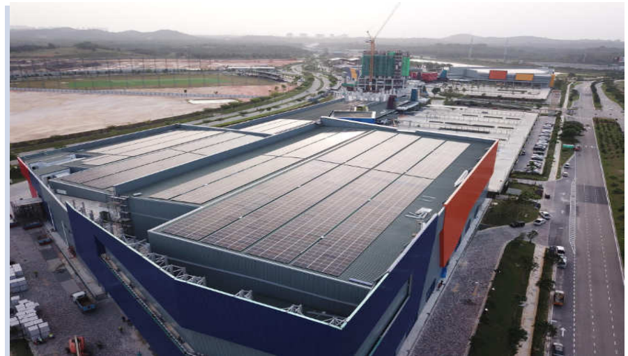
Roof Top Solar – Sunway Iskandar
