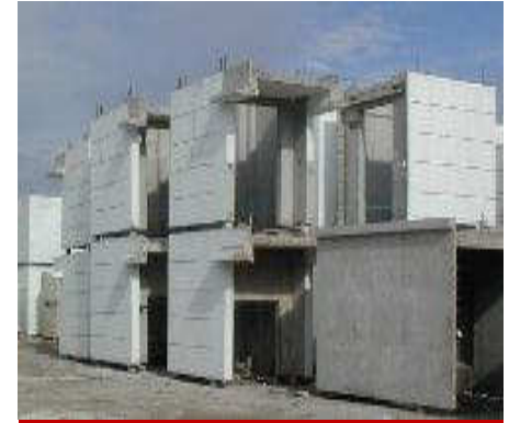
Lift Core Wall
