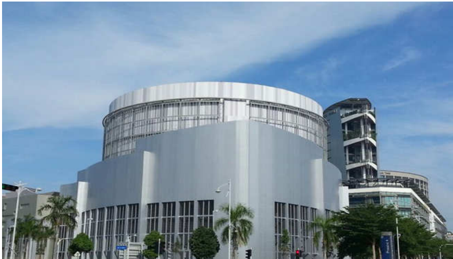
Gas District Cooling Plant - Putrajaya
